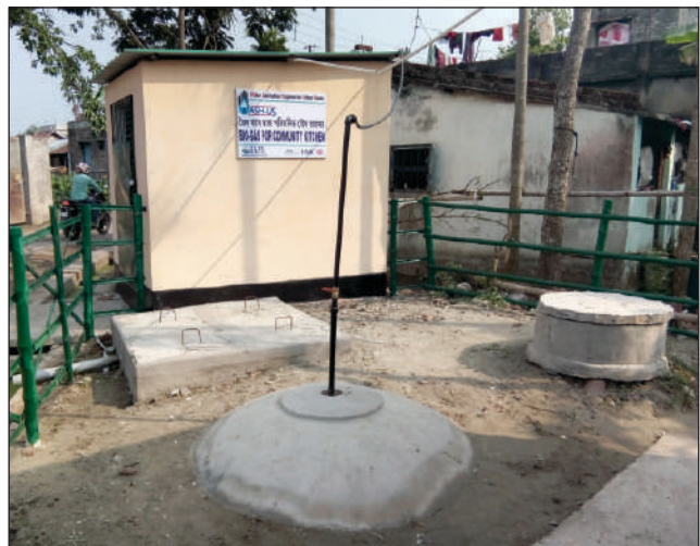
Bio-gas under construction at WASH-US site
